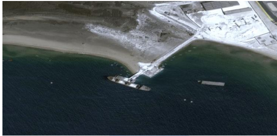
ABO ZNIMA PORT - SOUTH SINAIA, EGYPT.
